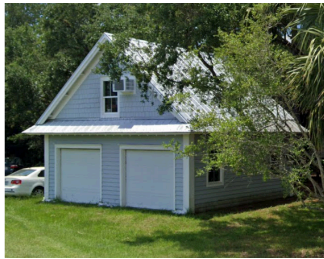
2 EXISTING GARAGE ADJACENT TO ION Scale: 1/8" = 1'-0"
