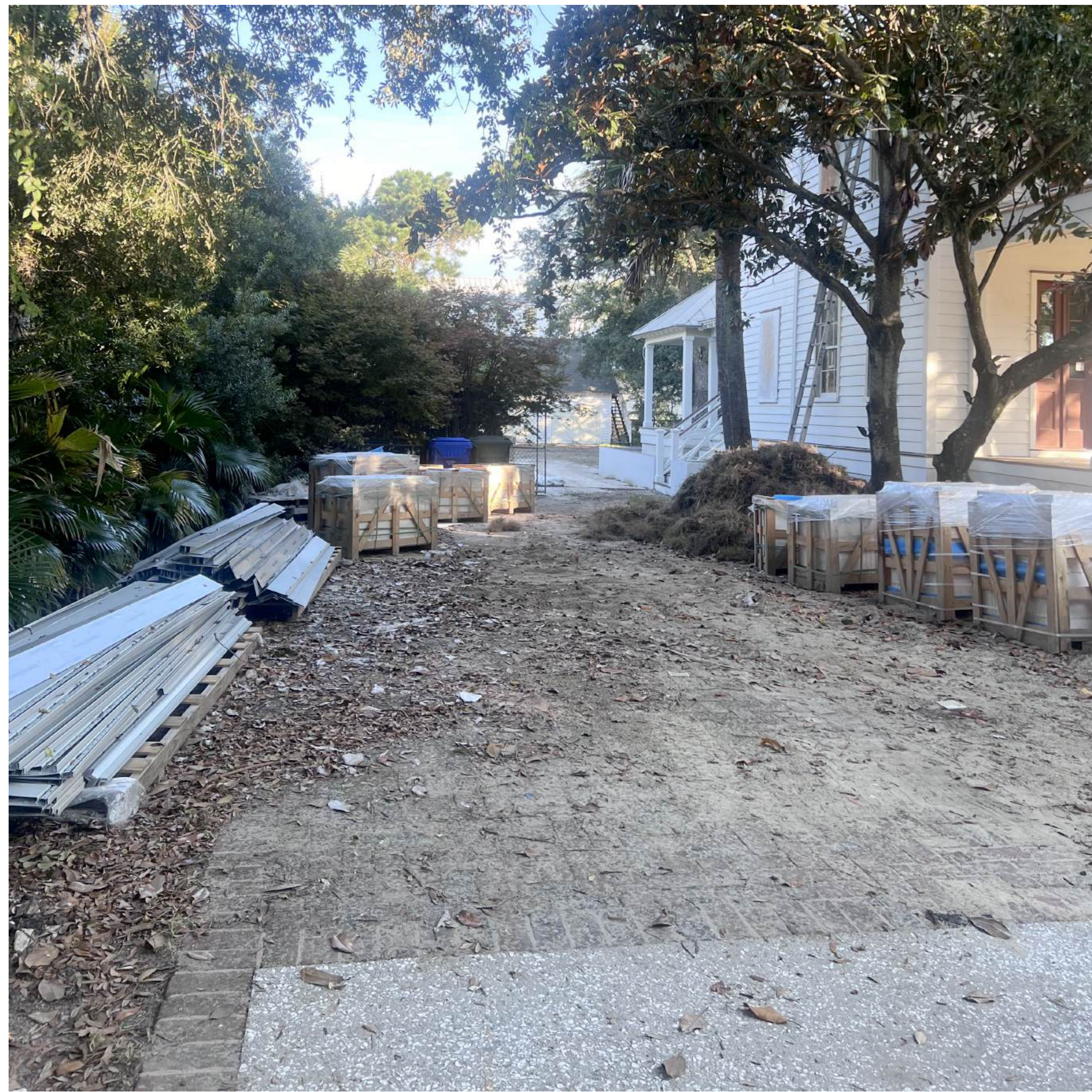
VIEW OF GARAGE FROM STREET
