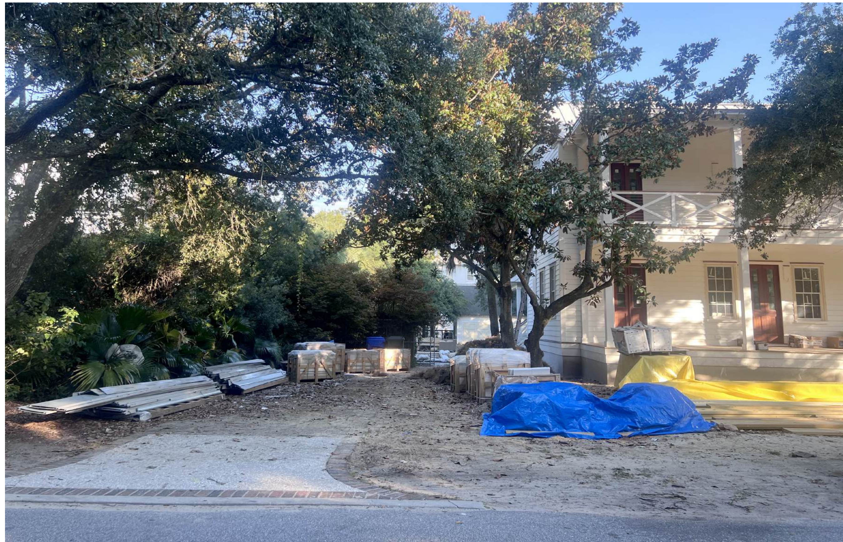
VIEW OF GARAGE FROM STREET
