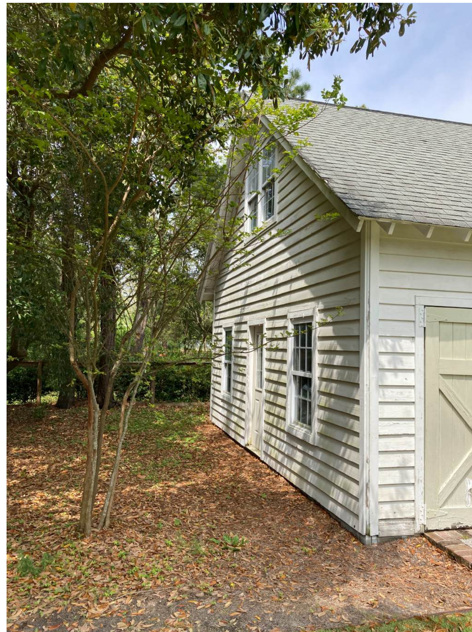
WEST ELEVATION OF EXISTING GARAGE
